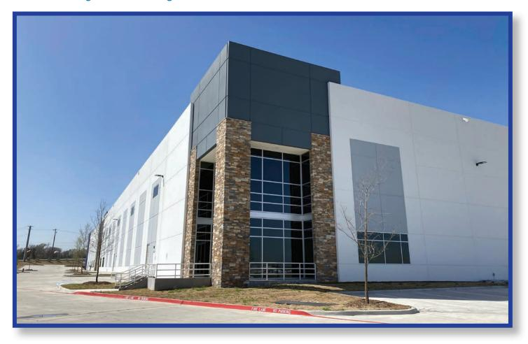
A cross-dock, 1,013,833 SF building designed and constructed by Commerce Construction Co., L.P. featuring a 40 ft clear space at first interior column line, ESFR fire sprinkler system, 50 dock leveler packages, and design build tenant improvements based upon tenants needs.
