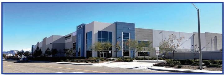
Design and construction of 600,000 SF concrete tilt-up building with on and off-site utility improvements including on site 130 KW Generac backup generators for Living Spaces.
