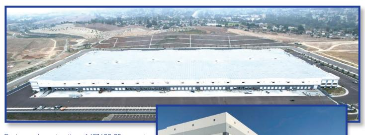
Design and construction of 627,480 SF concrete tilt-up building with on and off-site utility improvement including on site 400 KW Genset backup generator for FedEx Ground.
